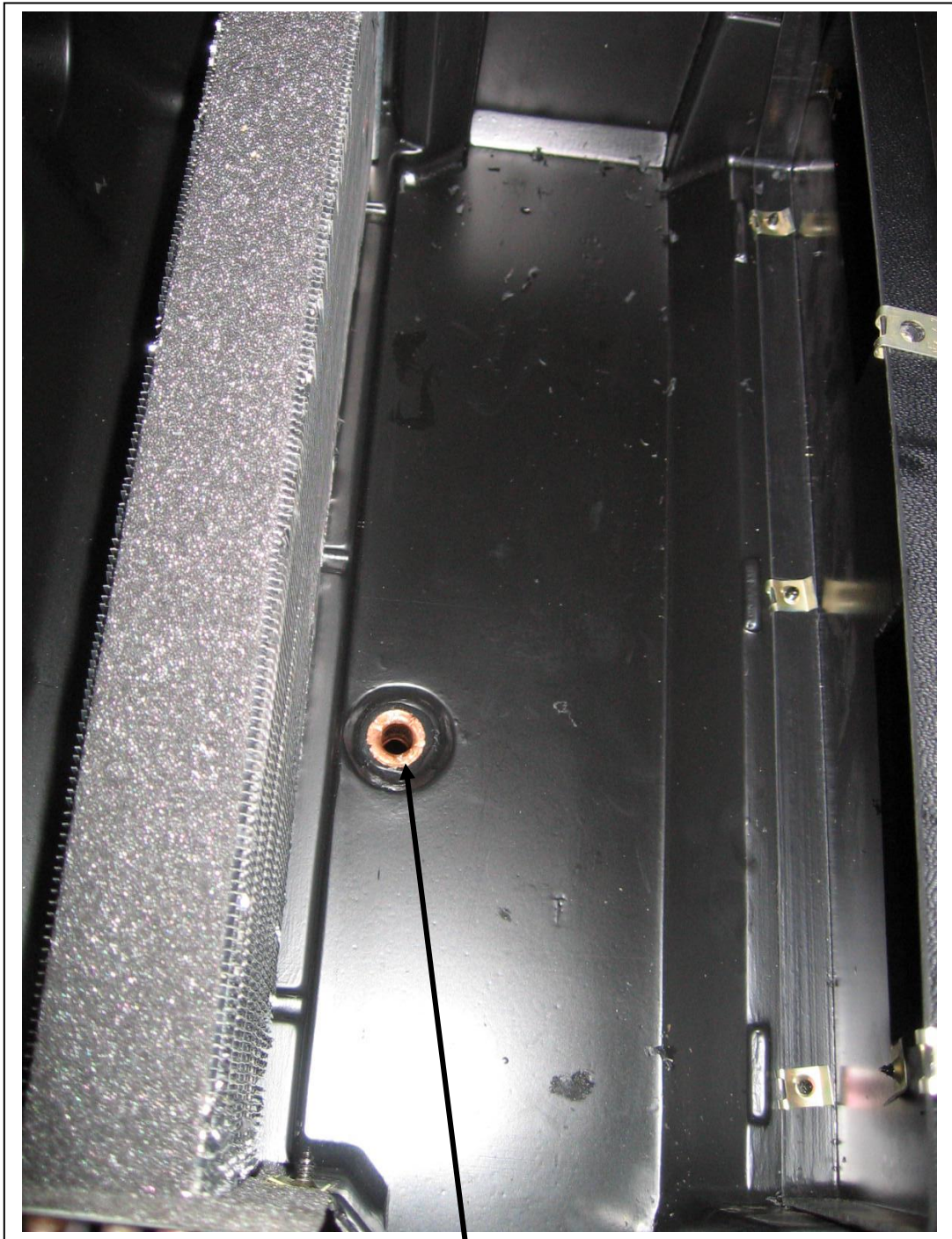
Copper glue in drain tube adapter in place.
